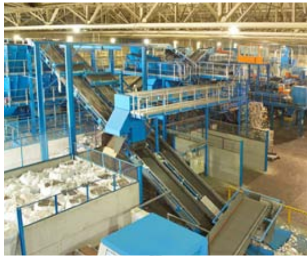
Above. AWS plastic reprocessing facility, UK.
