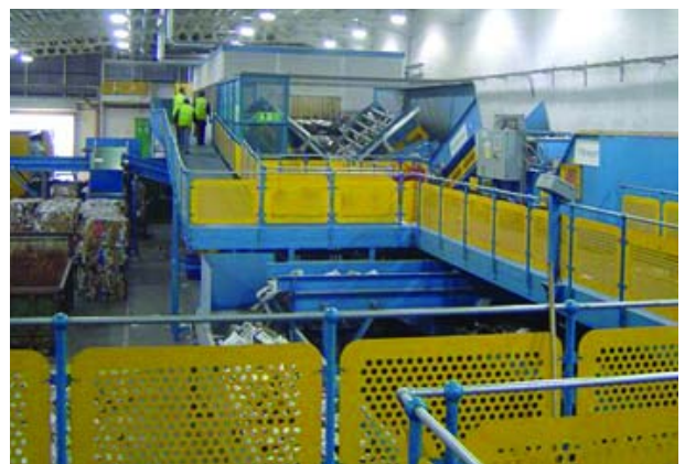
Material Reclamation Facility (MRF)
